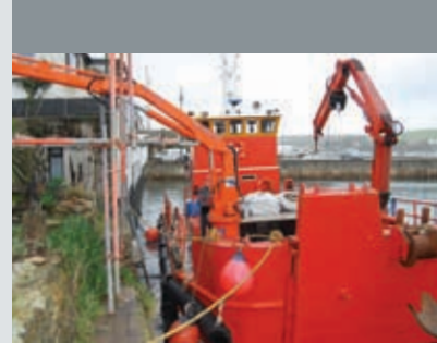
▲ Unloading 20 tonnes of building materials
