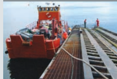
▲ Slipway repairs for the RNLI
