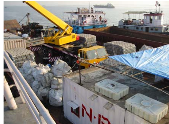
Concrete mattressing, India
